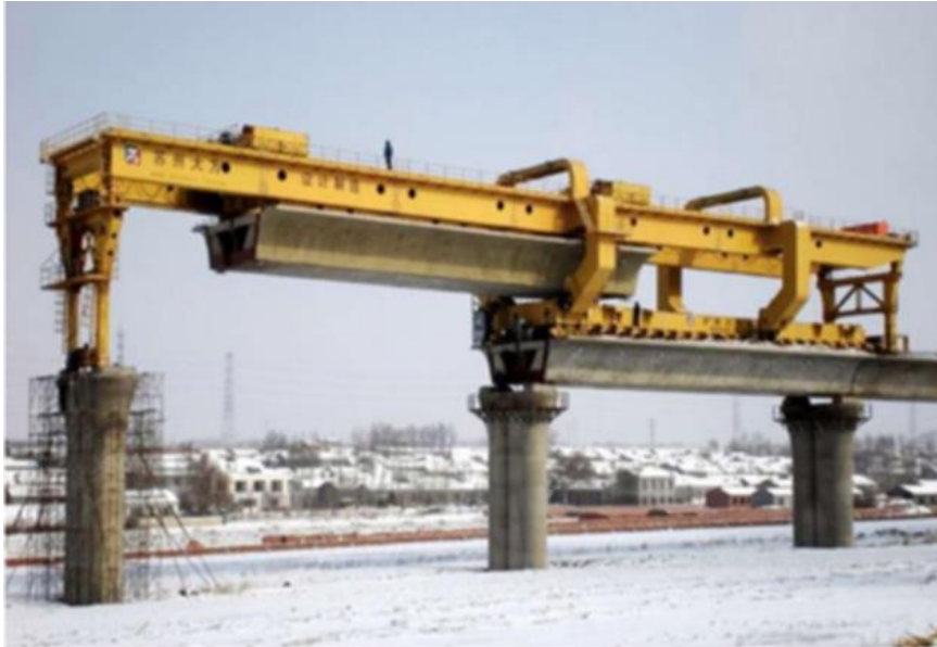
Figur 28 : Segmental bridge launching machine
