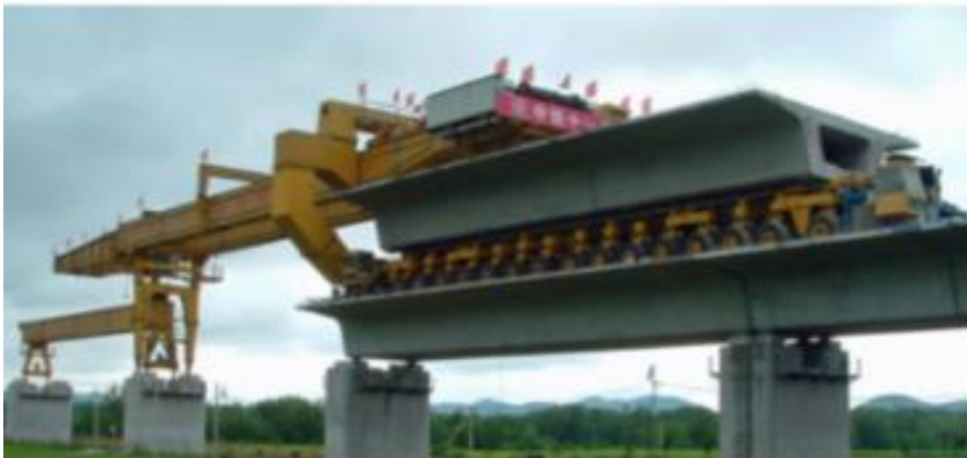
Figur 29 : Segmental bridge launching machine
